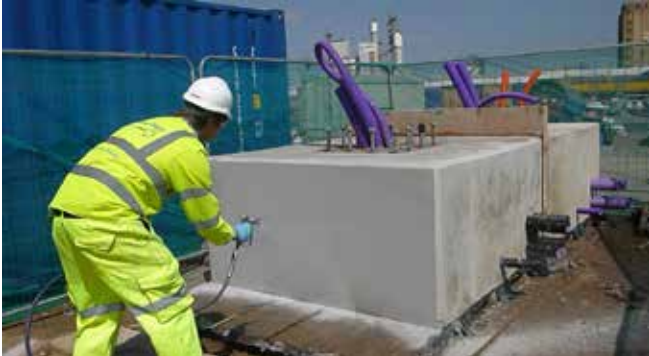
Intercrete 4841 effectively reinstates cover and protects from chlorides
