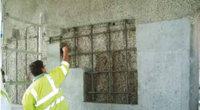
Intercrete 4800 can be applied up to 80mm thick in a single layer
